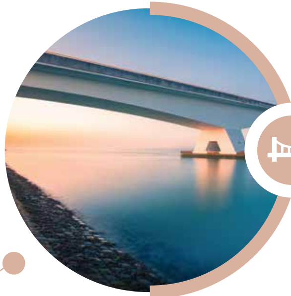
MMRDA Bridge to start from Ghatkopar and end at Kopar Khairane
